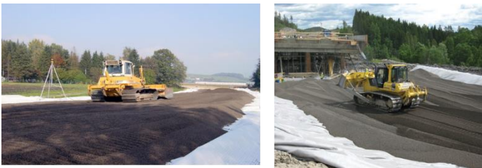
Figure 5: Bulldozer installation
