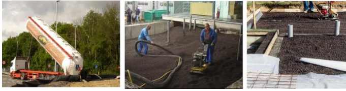
Figure 3: Blowing and vibrating plate levelling-compactation installation
