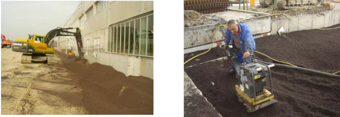
Figure 4: Excavator & vibrating plate levelling-compactation installation
